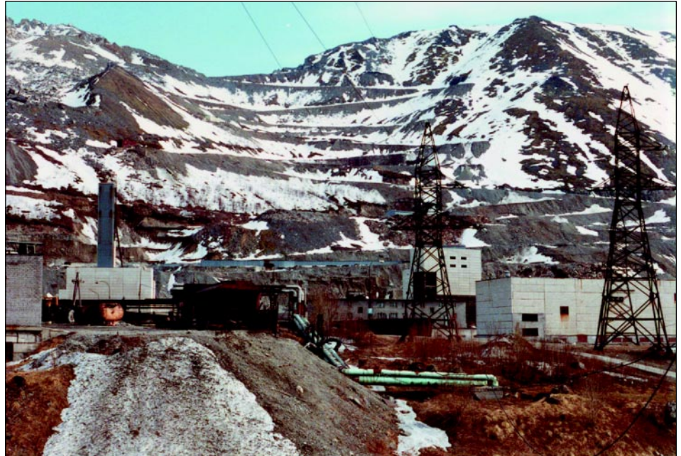
This apatite mine in Kirovsk is the world's largest source of apatite ore, which is crushed and exported to the south as a phosphorus source for fertilizers. The copious dust produced in the mining and crushing processes is a serious health hazard for the 115,000 people living in Kirovsk and Apatity (photo by Rasmus Ole Rasmussen).
